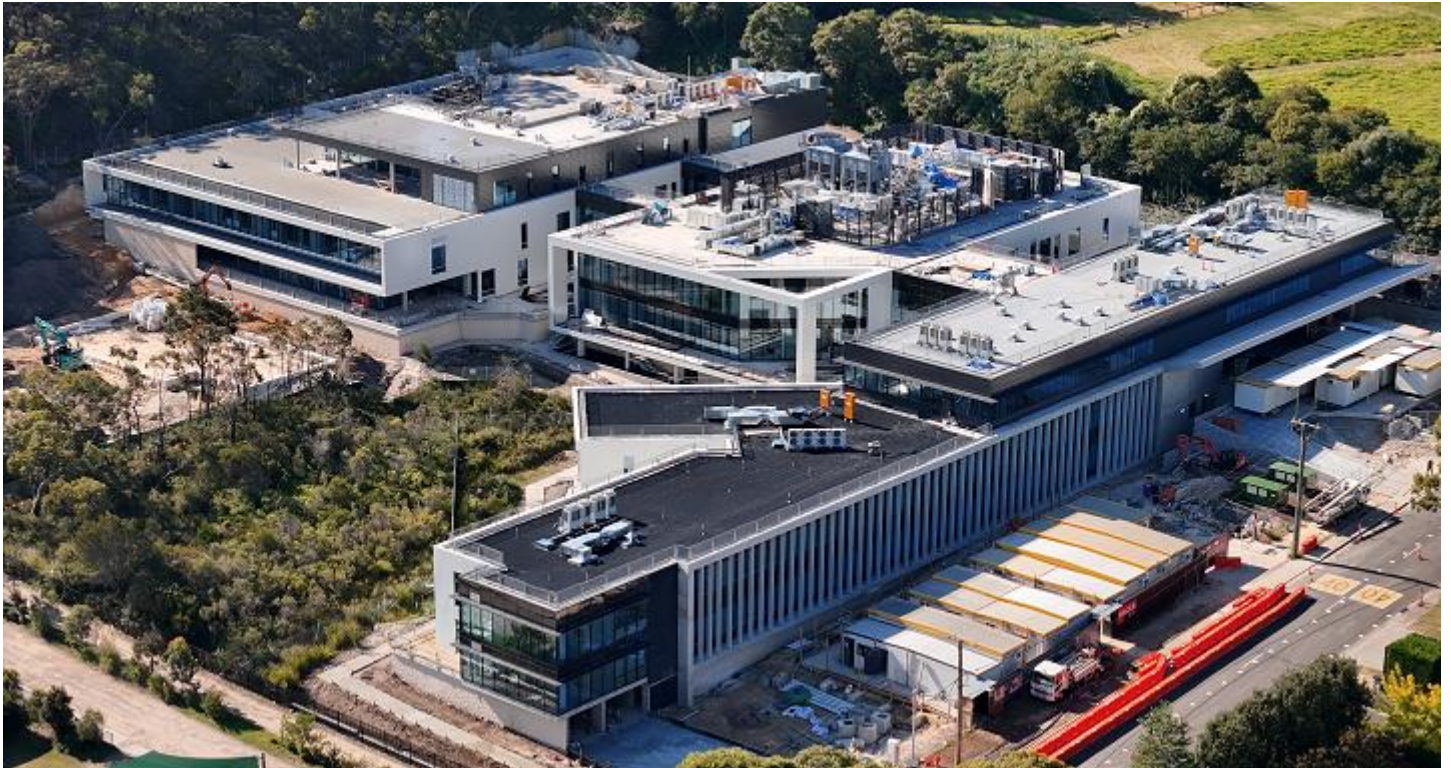
Wyvern Private Hospital (under construction), Terrey Hills, NSW
