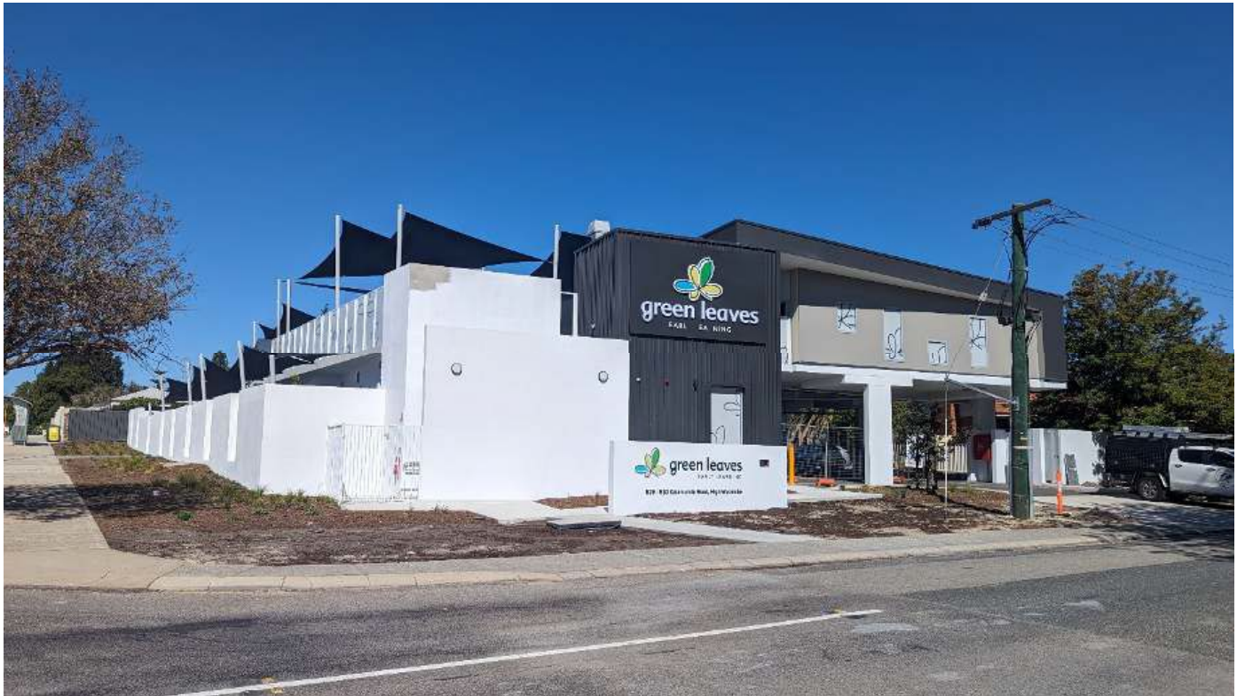
Picture: The Childcare Property Fund's latest development at 531 Kalamunda Road, High Wycombe, WA nearing completion.
